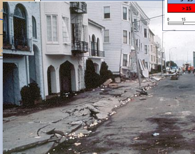
Liquefaction in San Francisco Marina, Loma Prieta Earthquake 1989
